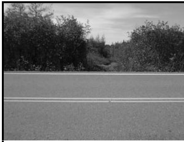
It is only a cut survey line right now, but this is where our new road will end.
